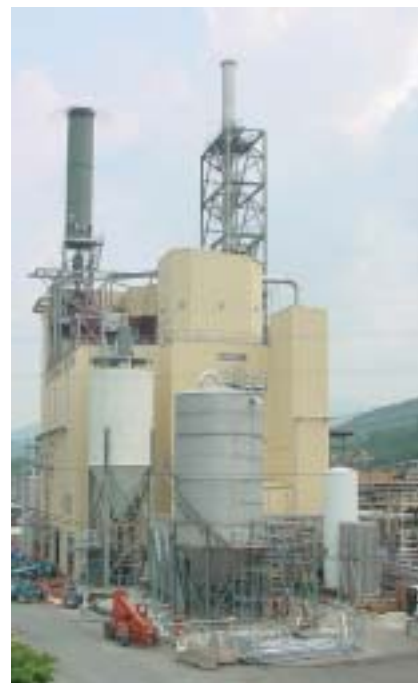
Black liquor gasifier at Georgia Pacific’s Big Island, VA pulp mill.
